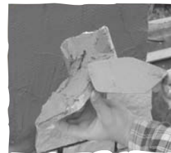
PHOTO 3 - Application of mortar onto Natural Thinstone Veneer
