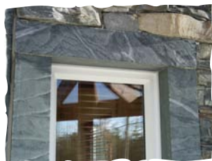
UPRIGHTS AND LINTELS
