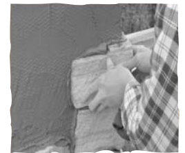
PHOTO 4 - Application of Natural Thinstone Veneer
