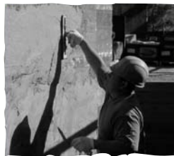
PHOTO 2 - Application of scratch coat to surface of exterior wall
