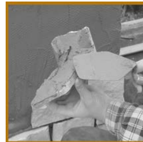
Application of mortar onto Natural Thinstone Veneer.
