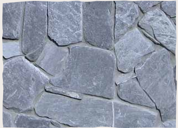
TOFINO SKY FIELDSTONE - MORTAR JOINT
